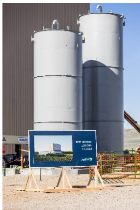
도표 4. Sodium Test and Fill Facility(2)
